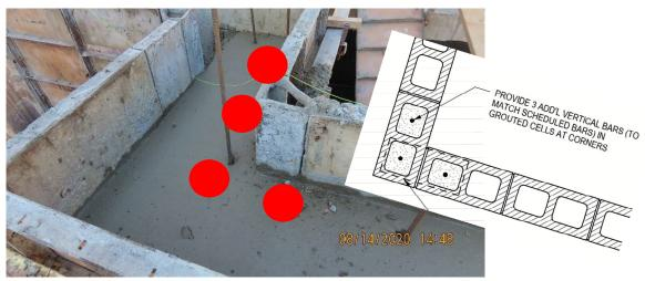
Missed and Mis-Located Masonry Rebar at the Corners
