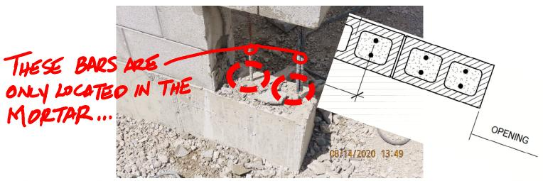
Concrete Rebar was missed and NOT Installed in the concrete and the Mason did not post install them...
